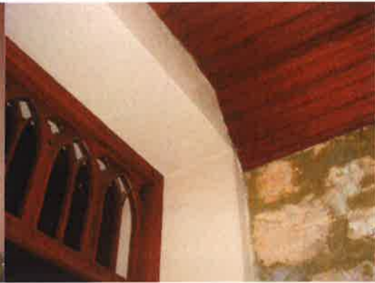
Photo 43: Detail of screen, stone walls and boarded ceiling
