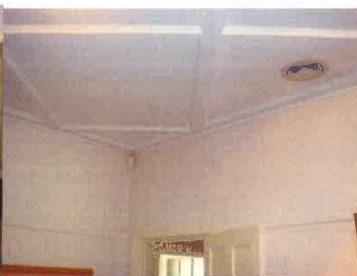
Photo 114: Dining room ceiling
