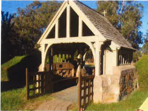
Photo 58: General view from east
