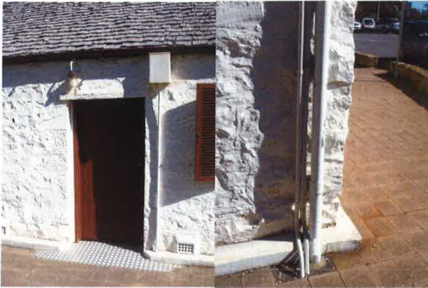
Photo 78: East door and steel access threshold
