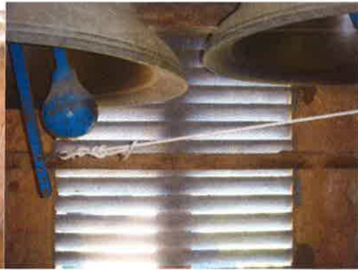
Photo 55: Belfry showing bells and timber louvres
