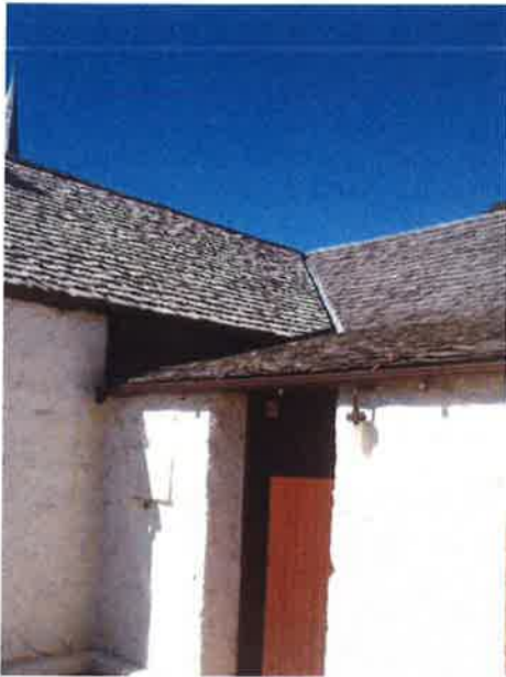
Photo 84: North side skillion and back door
