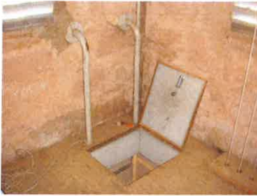
Photo 54: Belfry access hatch
