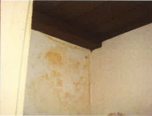
Photo 126: Water damage in Bed 3 closet
