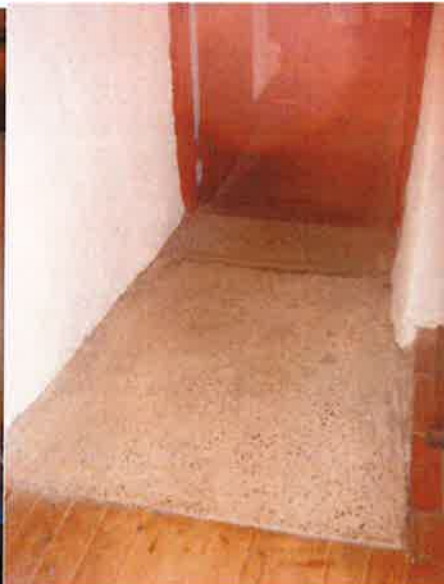
Photo 89: Concrete ramp in Room 2
