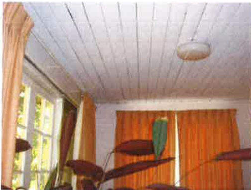
Photo 115: Enclosed verandah off Dining room
