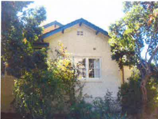
Photo 101: South side, living room window
