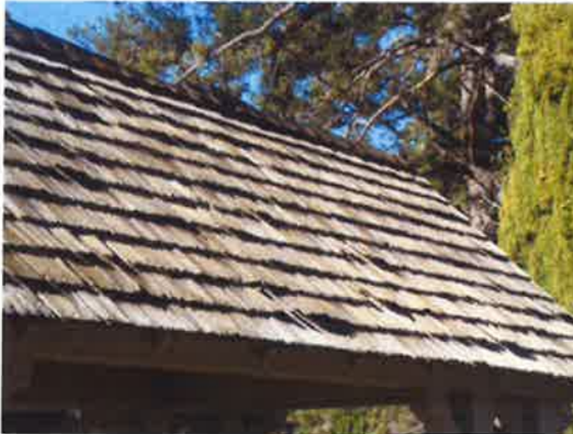
Photo 68: Detail of weathered shingles
