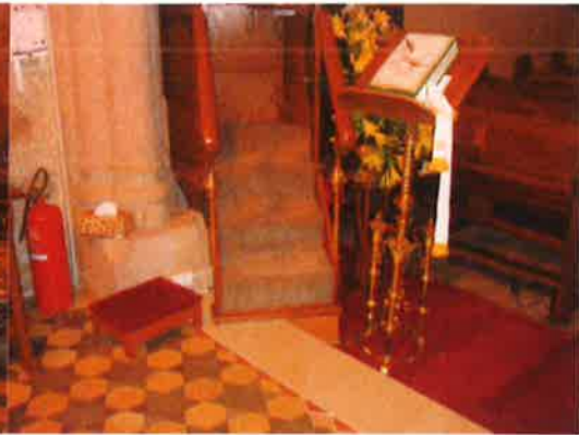
Photo 38: Pulpit and recently replaced stone step tread below Chancel arch.
