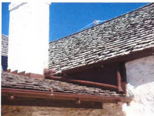
Photo 82: Close up of roof junction north side
