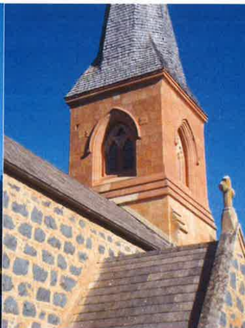
Photo 4: Detail of north porch roof and west tower
