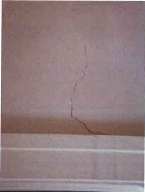
Photos 127 & 128: Typical cracking on internal walls
