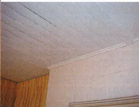
Photo 120: Main bedroom ceiling (formerly a verandah)
