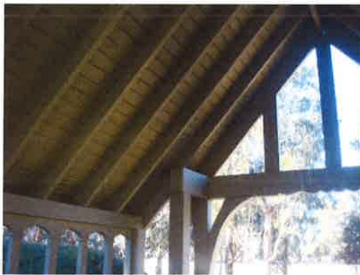
Photo 60: Detail of timber structure
