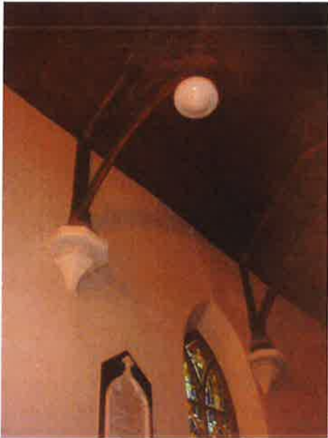
Photo 34: Upper walls of Nave
