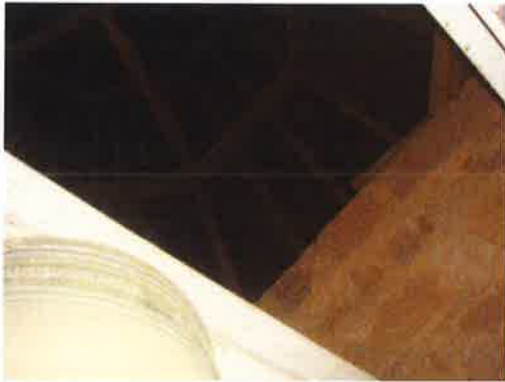
Photo 56: Belfry looking into roof area
