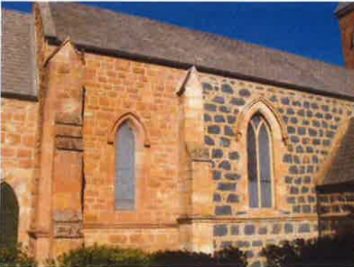
Photo 7: Detail of 1872 Nave extension
