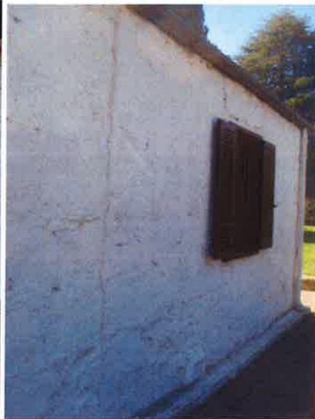
Photo 77: Line indicates the junction of the original 1845 building and the 1864 addition
