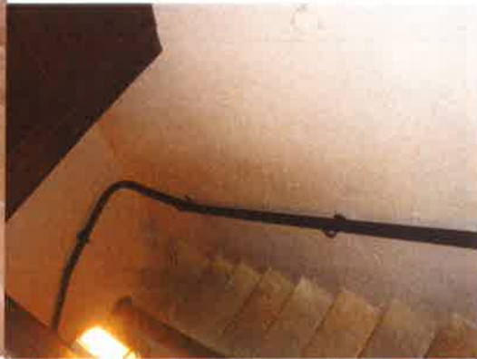
Photo 47: Stair showing stone steps and handrail installed in 2010
