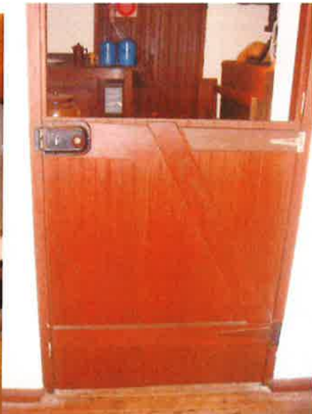
Photo 95: Typical internal stable door
