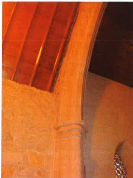
Photo 40: Chancel arch. Note the differing wall finishes
