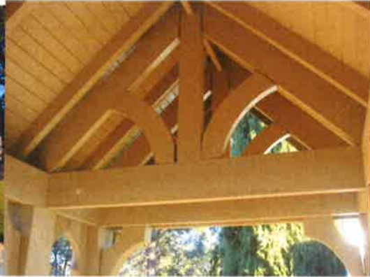
Photo 67: Detail of timber structure
