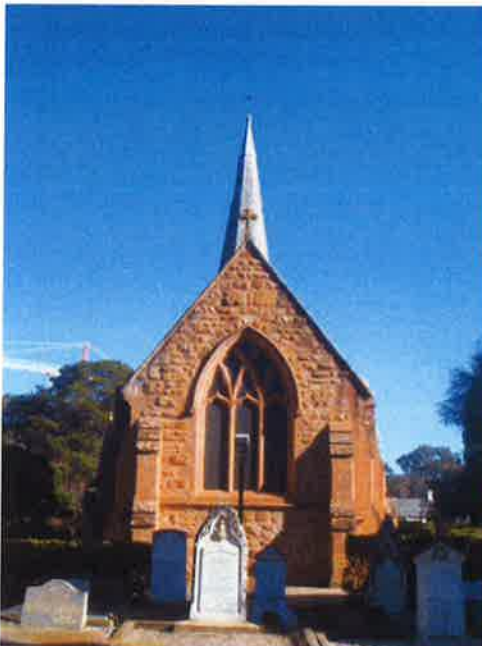
Photo 3: East side showing three part Gothic arched window
