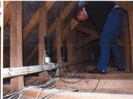
Photo 57: Church roof space
