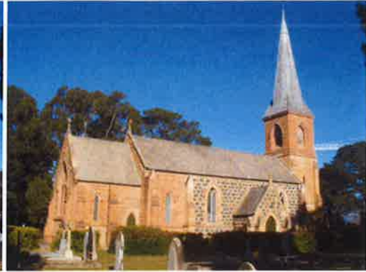
Photo 6: North elevation showing the different types of stonework
