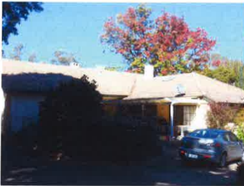
Photo 103: View from northwest
