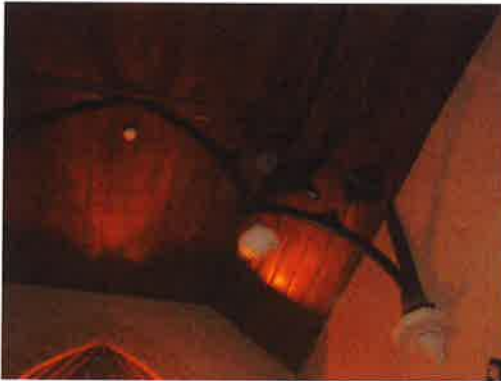
Photos 32 & 33: Ceiling detail showing corbels, trusses and timber lining
