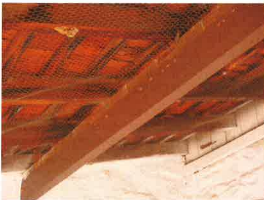
Photo 80: Exposed roof timbers north side porch window
