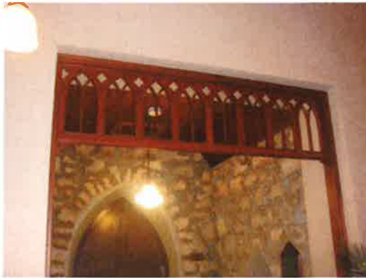
Photo 42: North Porch showing stone walls and fretwork screen
